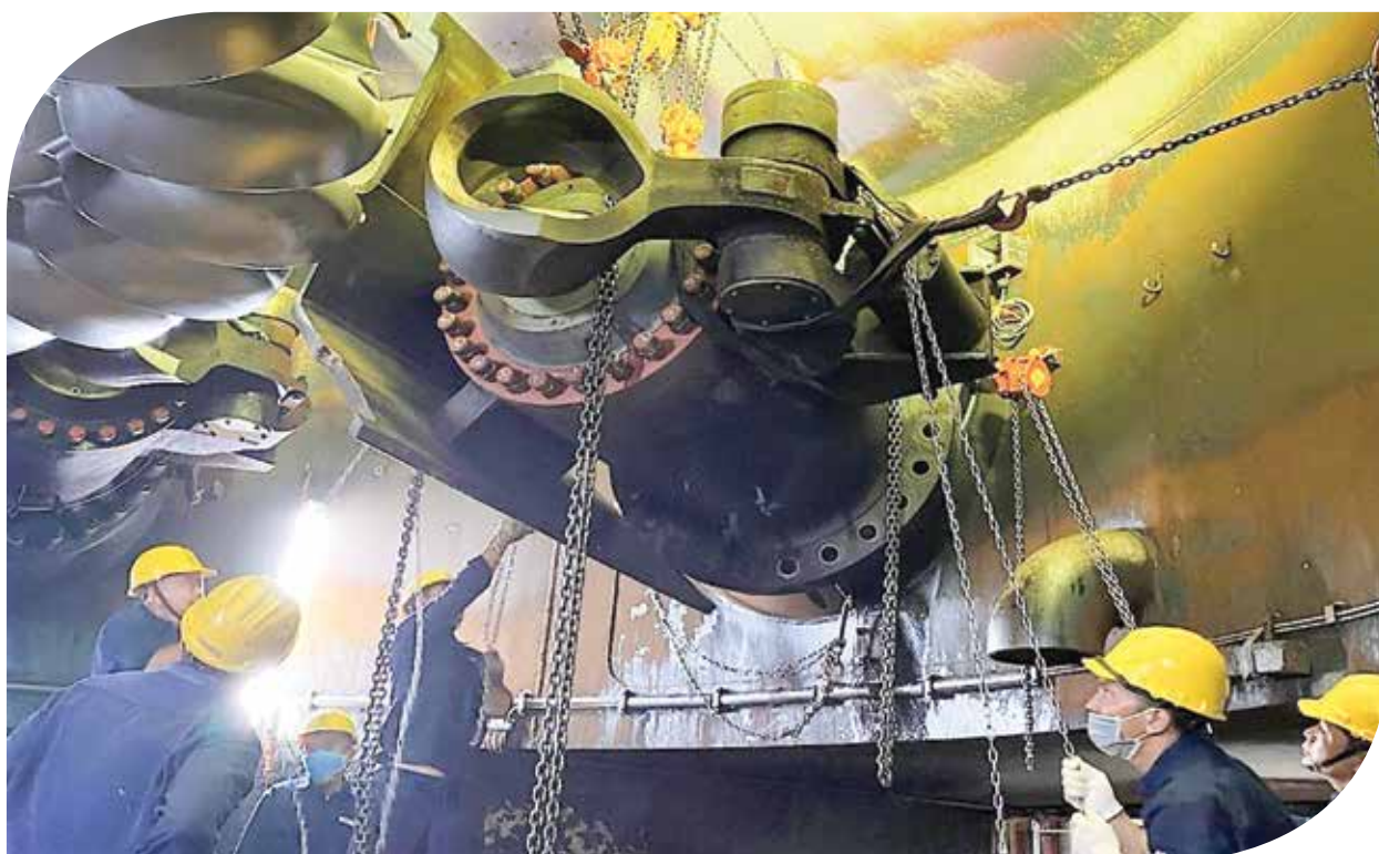
Repairing injectors at Dai Ninh Hydropower Plant
